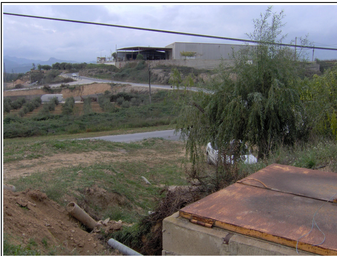
Vista general del pozo Aubals (05/01/2007)
